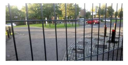
In order to prevent damage from strong wind, the cladding on the staff and traders' car park gate was changed from solid steel sheeting to 'paladin' type steel mesh. The effect of this has been to change the nature of the interface at this location such that some housing within Suffolk estate can now be seen from the Stewartstown
